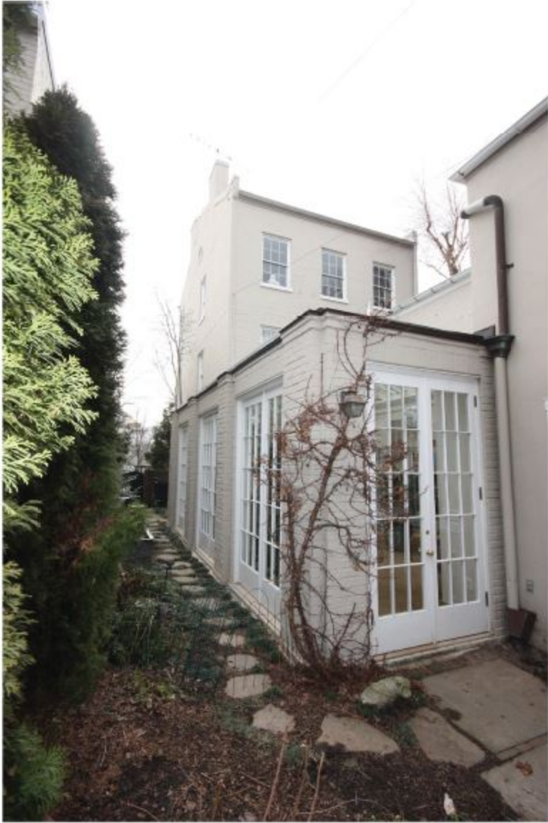
VIEW FROM NORTHEAST (BACK YARD)
