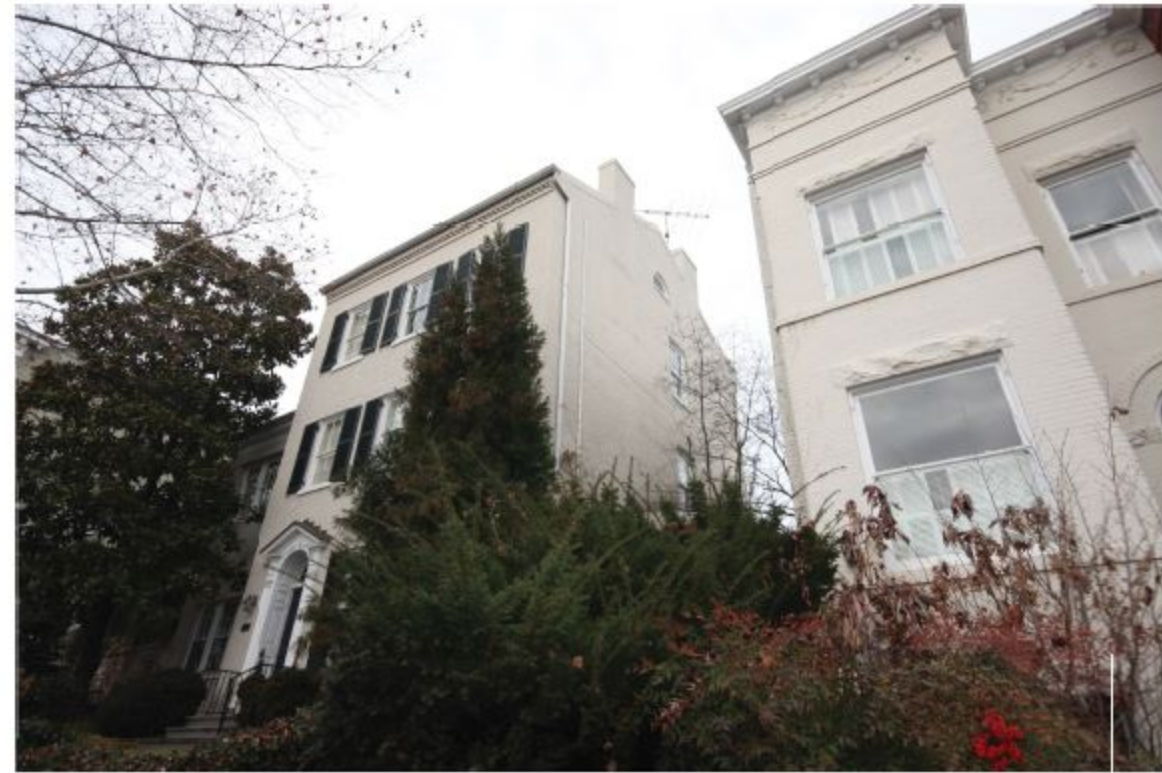
VIEW FROM P STREET (SOUTHEAST)
