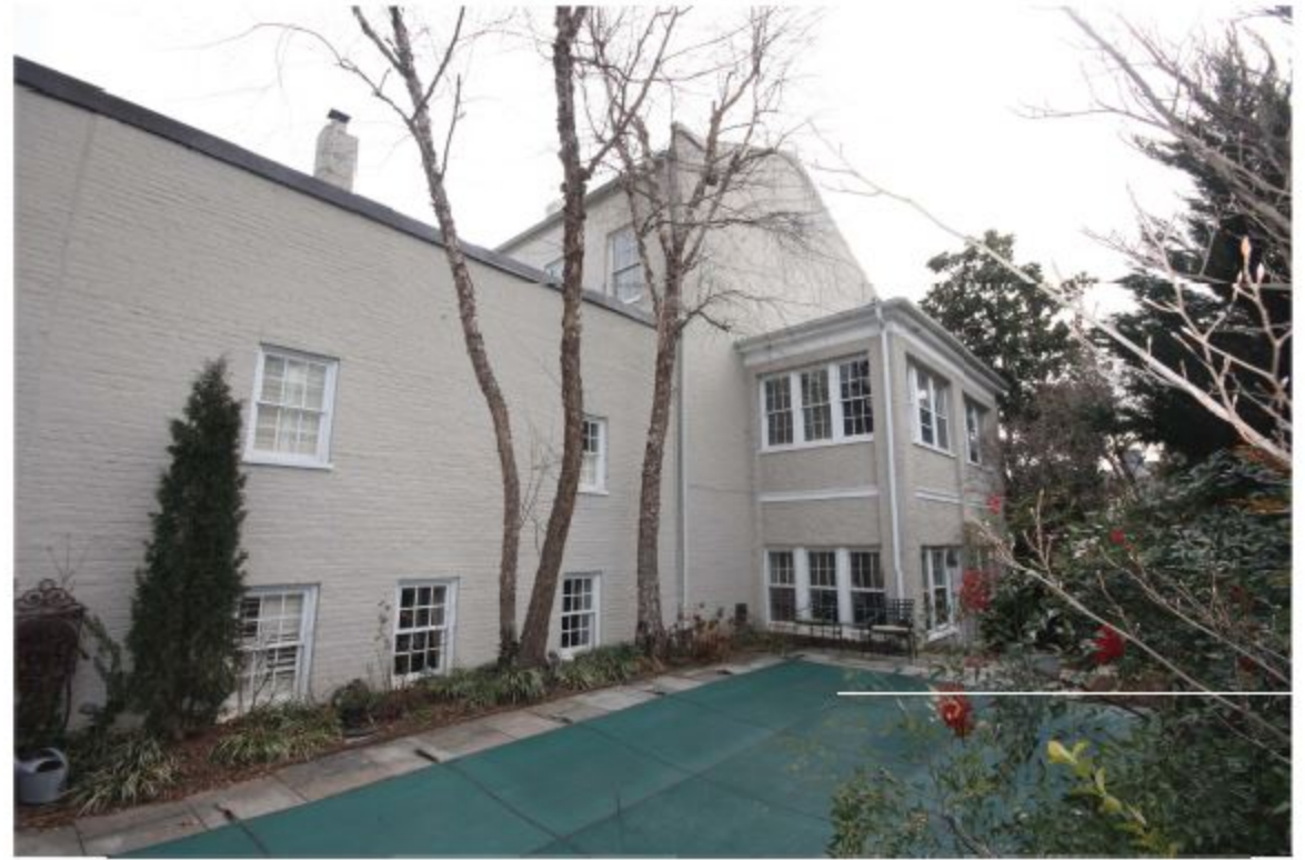
VIEW FROM NORTHWEST (BACK YARD)
